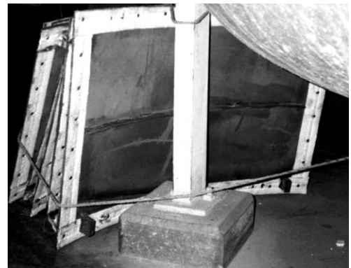
Loctite® 5920™ Copper securely seals pulverizer doors to prevent potential coal dust leaks, yet doors remain easily removable for service or inspection.
