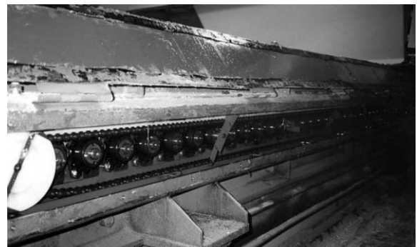
Loctite® 587™ Blue High Performance Silicone was able to seal the cover of the gear box on this Diamond Roll, eliminating oil leakage and associated labor costs.
