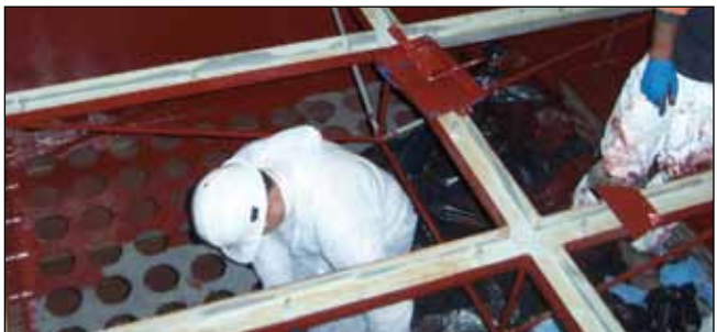
Applying Loctite® Nordbak® High Temperature Brushable Ceramic
