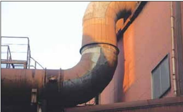
Plant pipe elbow, repaired with Loctite® Nordbak® Pneu-Wear
