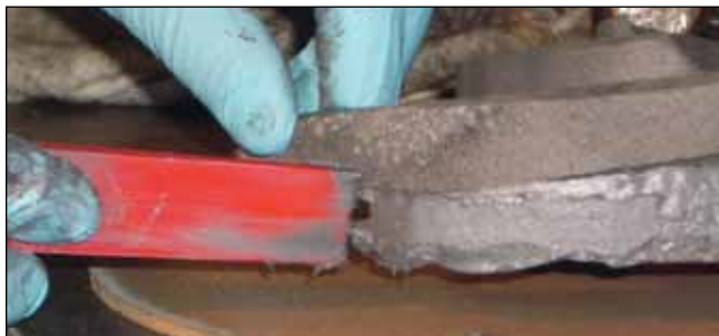
Repairing a pump impeller with Loctite® Nordbak® Wear Resistant Putty
