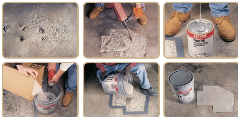
Your Source for FLOOR FILL Loctite® Fixmaster® Floor Fill 6-Step Process
