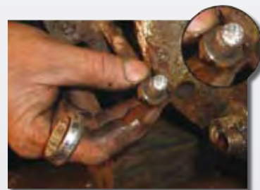
...which can lead to broken bolts.
